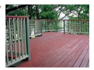
Although treated wood is protected against decay and termite attack, the application of a water-repellent sealer to all exposed surfaces is recommended when construction is completed. This sealer will help control surface checking (splitting or cracking) and provide an attractive appearance. Over time, reapplication of a sealer is recommended, perhaps every year or two.
