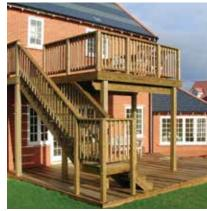
include a graspable handrail on at least one side. Railings must include a baluster system that prevents the passage of a 4-inch sphere. Refer to complete requirements and details for guards in the *Prescriptive Residential Wood Deck Construction Guide* (available at www.awc.org).
