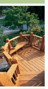
Decks and porches present a particularly severe exposure for both the wood and finishes. The horizontal surfaces, especially in decks, are often exposed to the direct rays of the sun and tend to collect moisture, therefore, the weathering process is greatly accelerated. As repeated cycles of wetting and drying occur, surface checks (small cracks) and end-grain surfaces begin to retain moisture.
