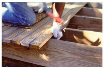
When installing the porch flooring material, begin with a coat of a mildew-resistant oil-based primer for exterior use applied to all four sides and the ends. Consider applying a coat of the final oil-based porch enamel to both the tongue and the grooves (also to the end of any piece that will be adjacent to the house) and installing it while the paint is still wet. This procedure not only assures an effective seal against moisture penetration, but also provides a good bond between floor boards.
