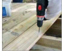
less corrosive overall than wood treated with dissolved copper preservatives, such as ACQ, CA and CCA. In addition, interior, dry environments are less conducive to corrosion than exterior, wet environments. Particularly severe environments include swimming pools, below-grade foundations, salt water exposure, trapped water and other environments that allow for constant, repetitive or long periods of wet conditions.
