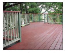
satisfactory long-term performance of pressure-treated decking is to minimize its dimensional changes. This can be accomplished by including a water repellant in the treatment process, drying after treatment and re-applying a water-repellant finish when needed. For additional information on finishing and maintaining decks, refer to the SFPA publication *Southern Pine Decks and Porches* and visit SouthernPineDecks.com.
