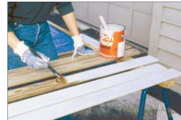
We applied the first coat of enamel before cutting the boards to length. This allowed the paint to dry while we built the frame for the porch. You can brush or spray the enamel. Wear gloves and work in a well-ventilated area.
