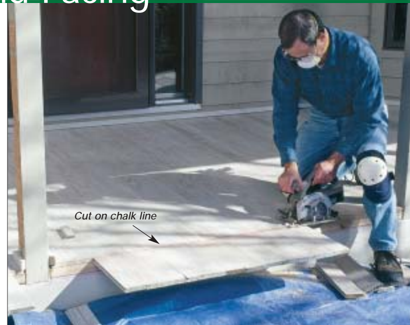
We notched some floorboards to fit around the porch posts and cut the rest to length after installation. A circular saw wouldn't cut up to the post, so we used an electric handsaw (left) to cut flush with the post and completed the cuts with a circular saw (above). Be sure to place a tarp beneath the cutting area so that you can collect and dispose of the sawdust safely.
