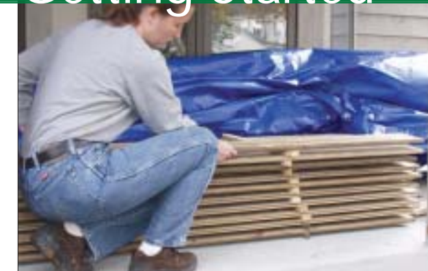
Stack the floorboards with stickers (spacers) to help them acclimate. Loosely cover the pile with a tarp to protect it from moisture. Be sure the pile is not in direct sunlight.
