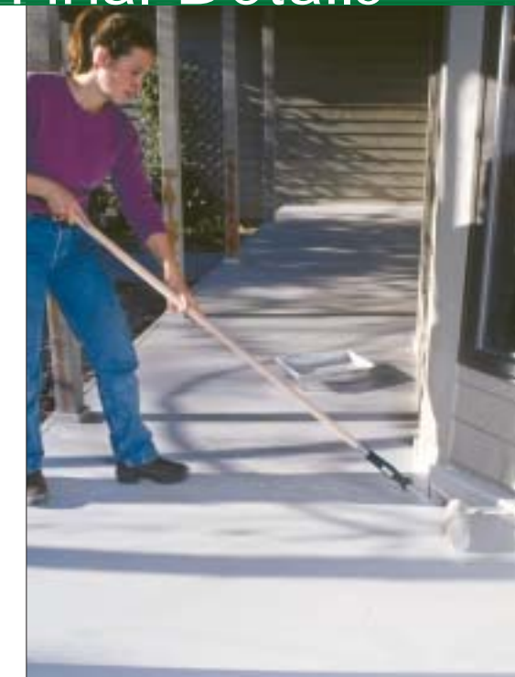
Use enough paint to thoroughly coat the wood. This protects it from weathering and provides a finished appearance. As we touched up the trim with a brush, we also coated the fasteners with paint.
