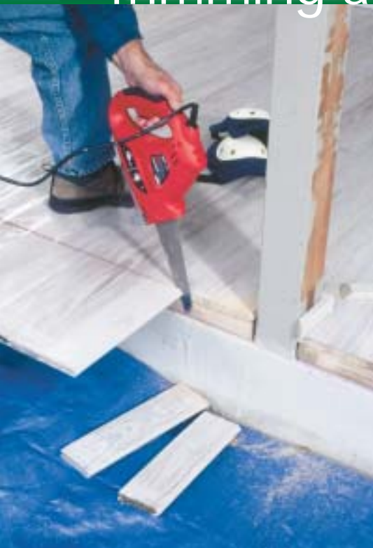
We notched some floorboards to fit around the porch posts and cut the rest to length after installation. A circular saw wouldn't cut up to the post, so we used an electric handsaw (left) to cut flush with the post and completed the cuts with a circular saw (above). Be sure to place a tarp beneath the cutting area so that you can collect and dispose of the sawdust safely.
